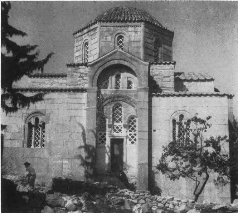
Εἰκ. 277-8. Ὁ ναὸς τῶν Καμπιῶν πρὸ καὶ μετὰ τὰς ἐπ' αὐτοῦ ἐργασίας.
