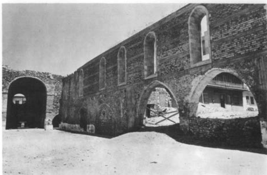
Fig. 7. Saint Peter Martyr. The nave.
