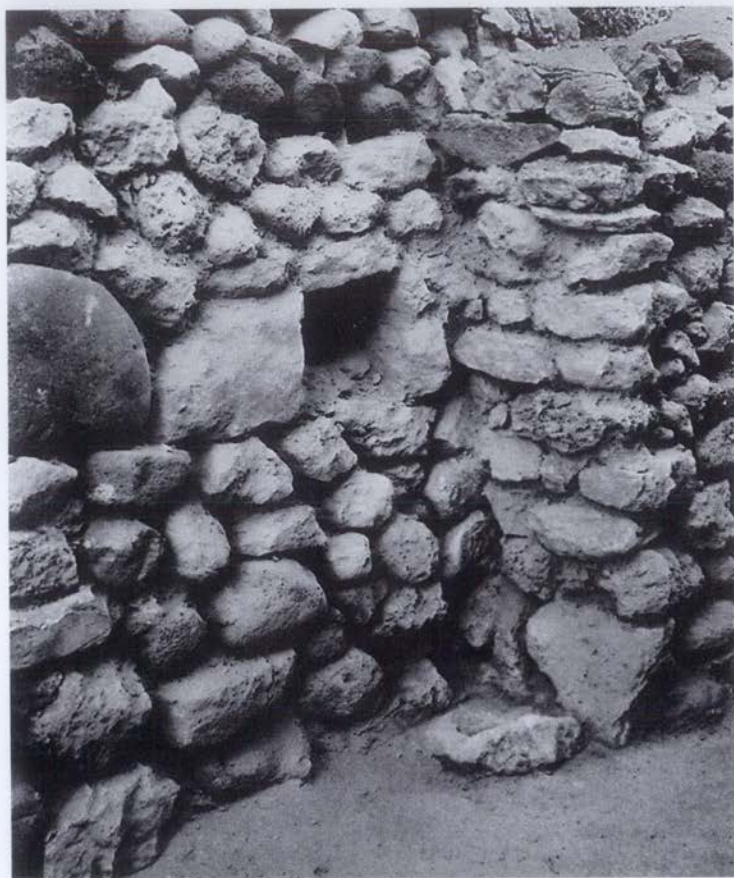
Fig. 84 Inside the gateway passage: left-hand gate jamb with opening for bolt; bottom: the gatepost socket.
