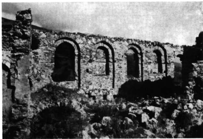
Εἰκ. 107. Σπίτι E. Ἐσωτερικὴ ὄψις τῶν καμαρῶν καὶ τῶν κογχῶν τοῦ κατὰ μῆκος τοίχου.
