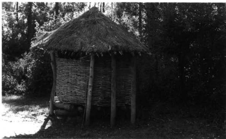
36. Similar storeroom in Kenya with a floor of tree trunks to prevent damp (photo 1988).
