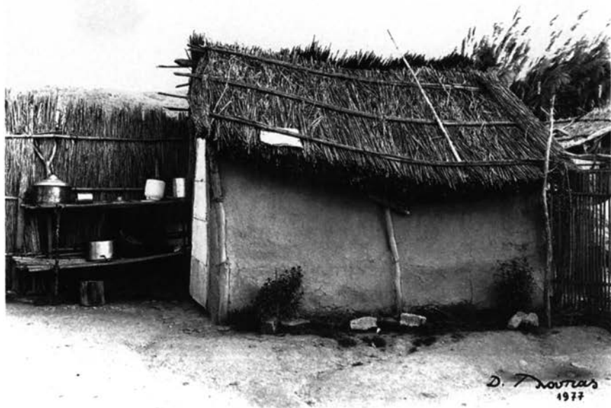
27. House in the district of Sykourio (Thessaly) with external struts for the thatched roof (photo 1977).
