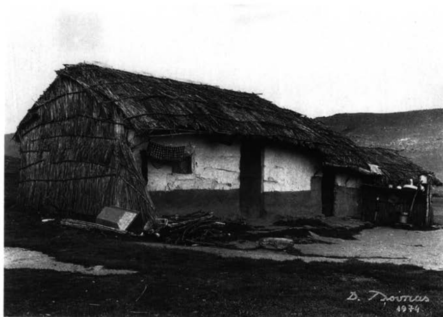
26. Mudbrick house in the district of Sykourio (Thessaly) with horizontal timbers built into the wall (photo 1974).
