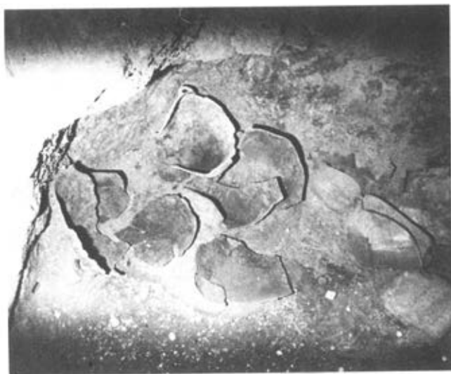
Fig. 12. Cutting in the rock near pillar No 7.
