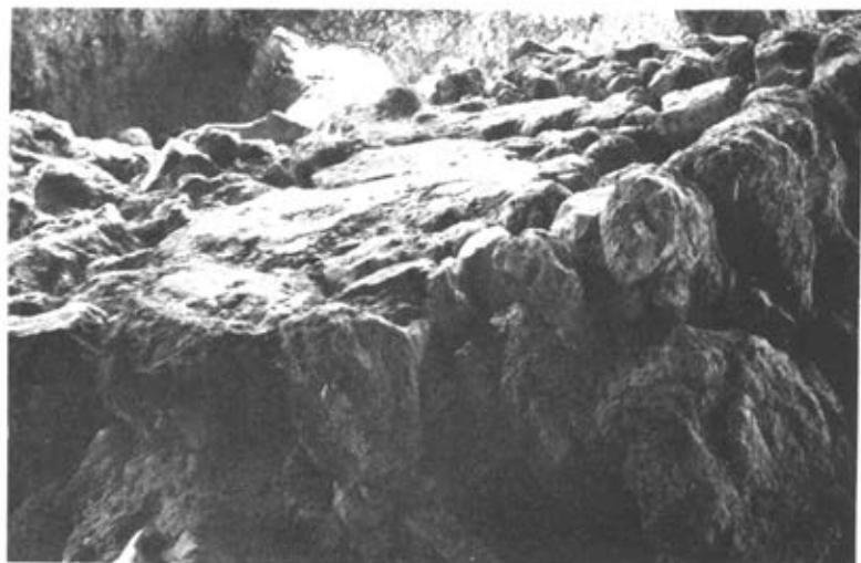
2. The fallen wall of the above picture still showing its plaster.
