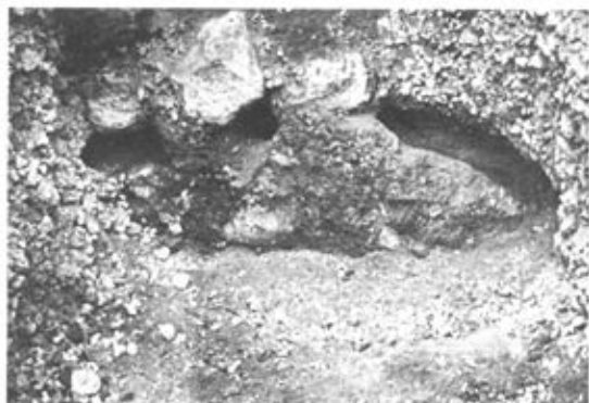
Fig. 56. The hollows of the wooden framework for the walls are instructive.
