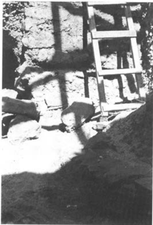
Fig. 21. Wall in reservoir trench, to North of shed in torrent bed.
