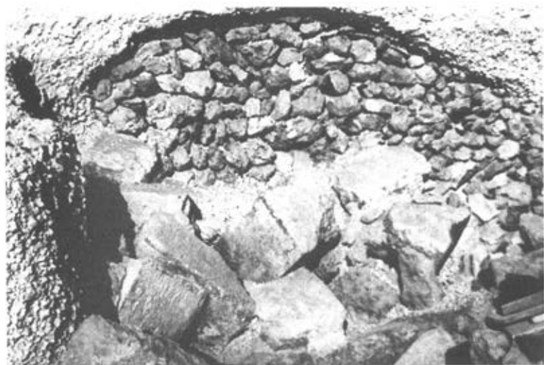
2. Area Γ'1 near pillar 4. Cavity in the pumice (walled by us for safety purposes).
