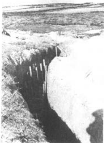
3. Drain coated with concrete.
