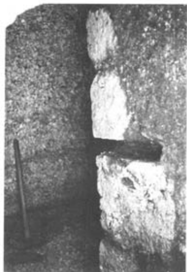
2. Tunnel. West House corner showing grooves left by wooden wall frame.
