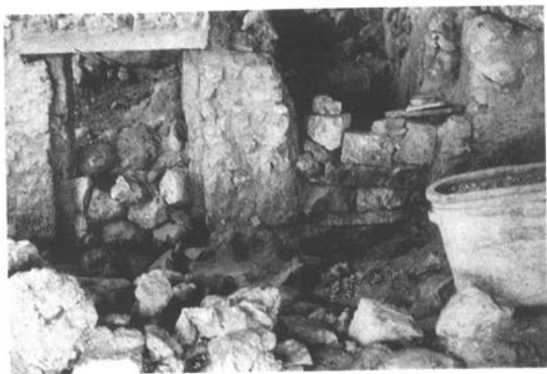
2. The walling of the doors by the squatters.
