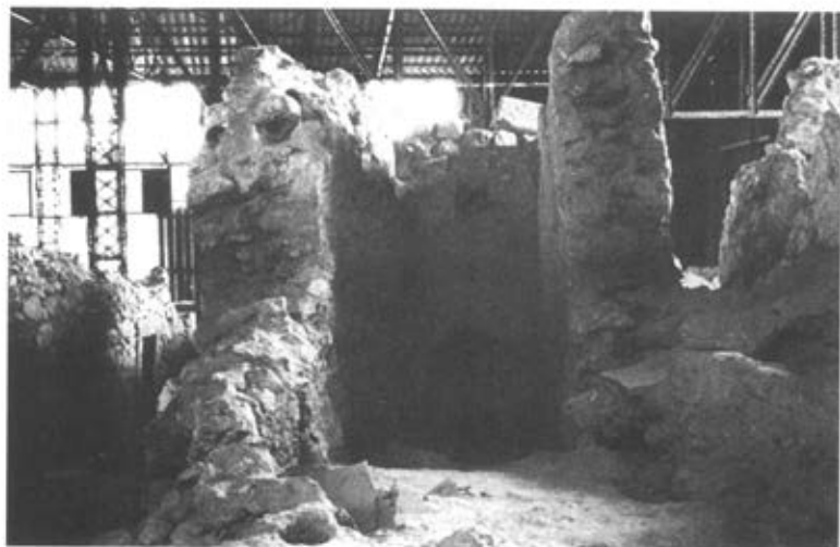
2. Corridor Γ5 in the centre; in the background a gap in the wall (possibly an entrance to the basement).
