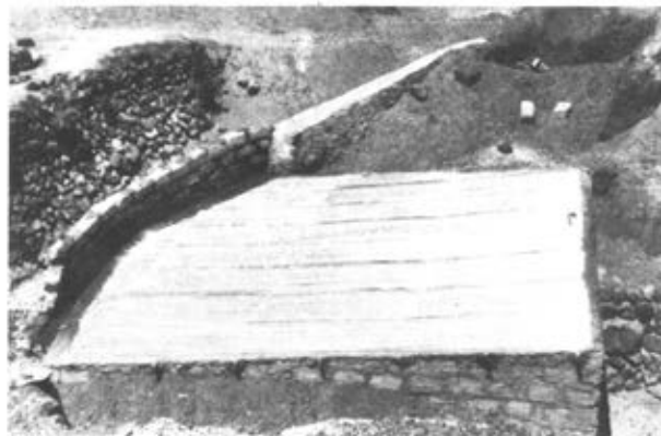
Fig. 43. The store-room was provisionally roofed to pass the winter.
