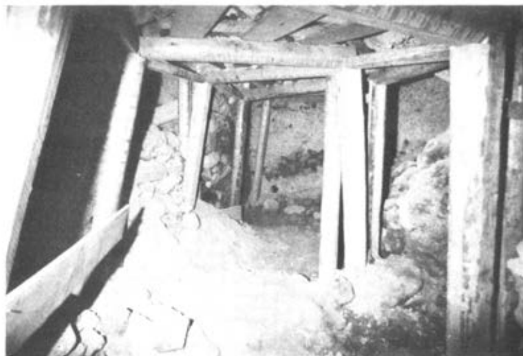
1. The tunnel of Quarter A.
