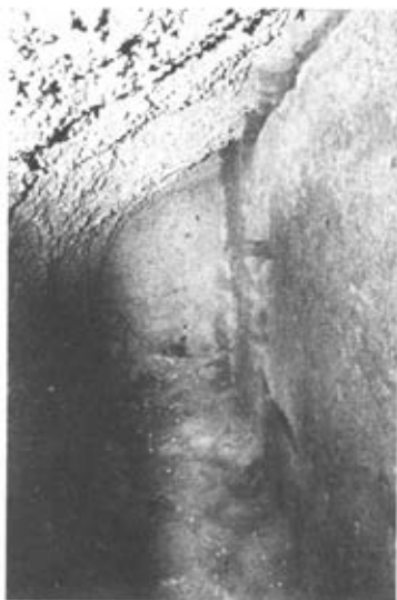
3. Tunnel. Innermost part showing wooden wall frame and window clearly on the wall.
