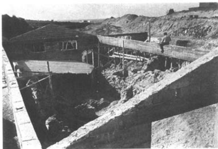
2. Shed of magazine Arvaniti 1 under construction.
