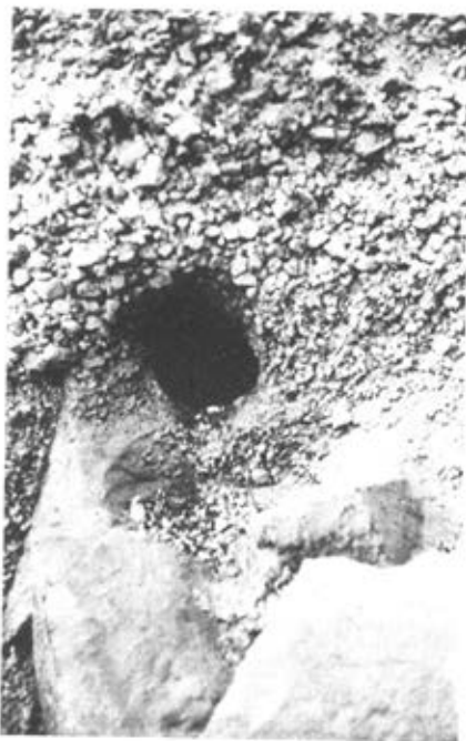
Fig. 23. One of the holes is rectangular in section, that is the beam was square.
