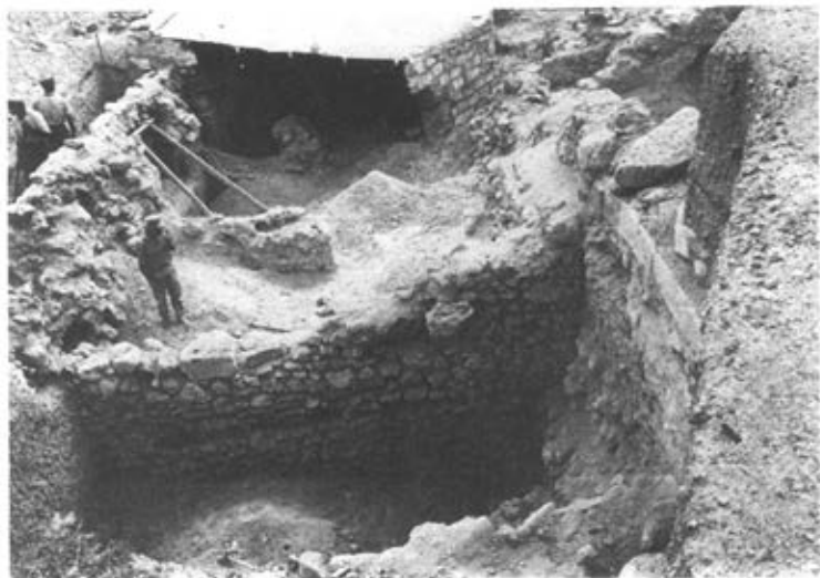
1. Arvaniti I. Magazine from North. Groove of horizontal beam of wooden wall-frame shown clearly on outer wall.
