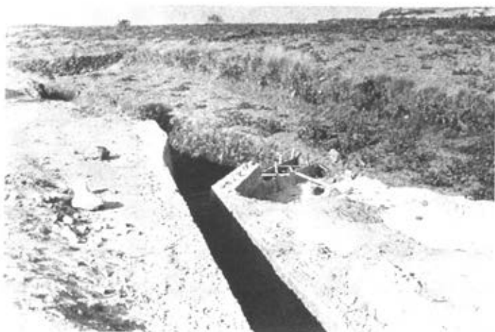
1. Arvaniti 1. Beginning of drain from South.
