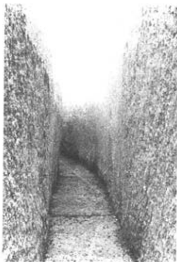
2. Drain from South.
