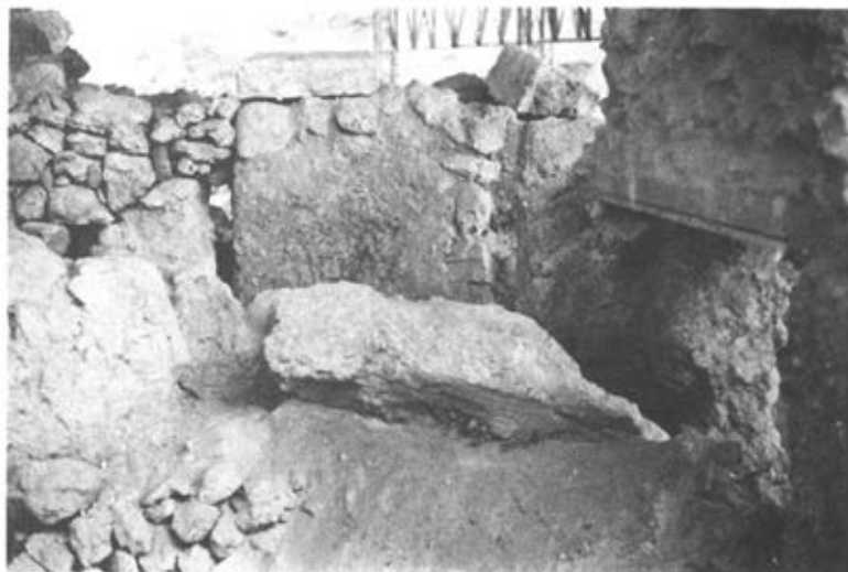
1. A fallen lintel of the door from Γ7 to Γ6.
