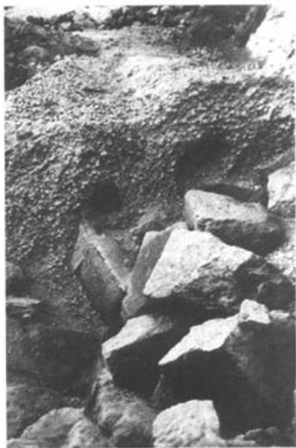
Fig. 22. Fallen stones and holes of beams in the pumice near pillar 4.
