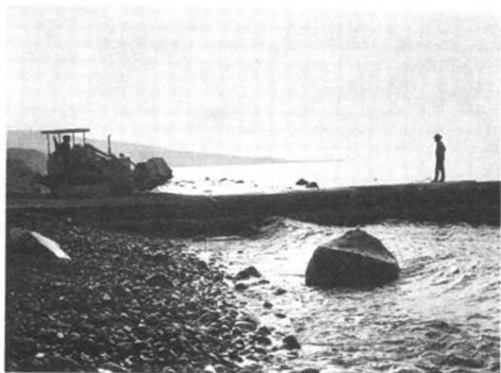
Fig. 30. A complementary technical work in 1969 was the construction of a mole for landing on the shore, near the excavation.
