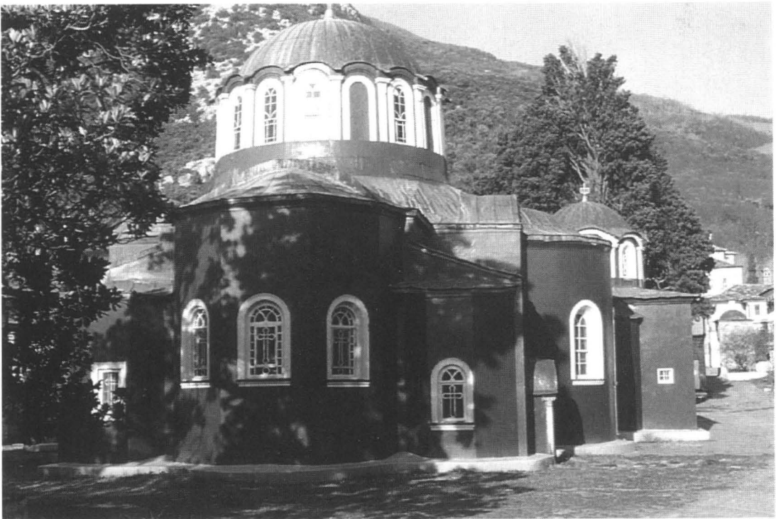
Fig. 18: Catholicon of Megisti Lavra Monastery at Mt. Athos, from the East.
